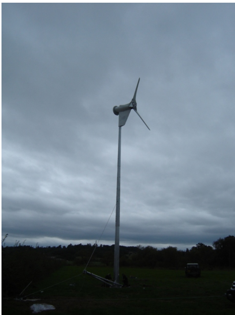
Typical Proven 6kW Wind Turbine.
