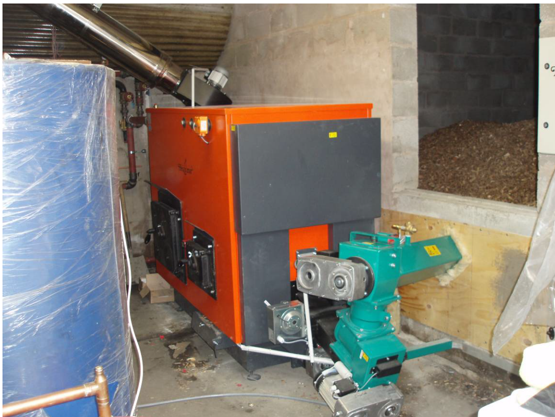
Typical wood chip boiler showing chip store
